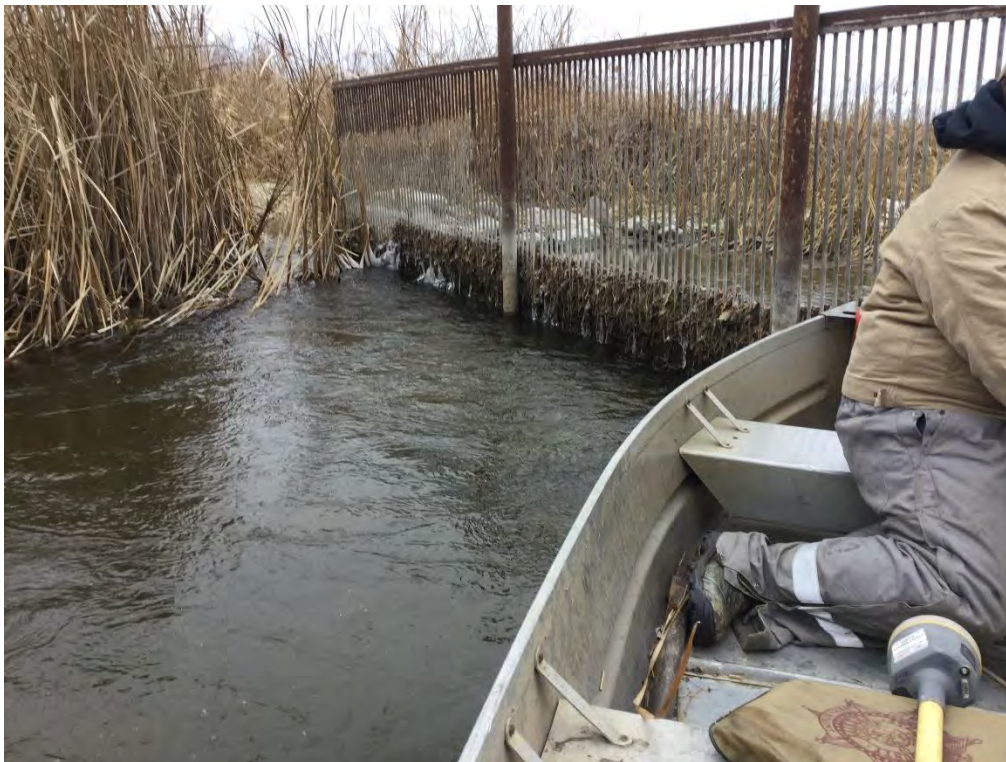
Photo 4: Fish barrier meeting the bank at the outlet of Two Rivers Lake.
