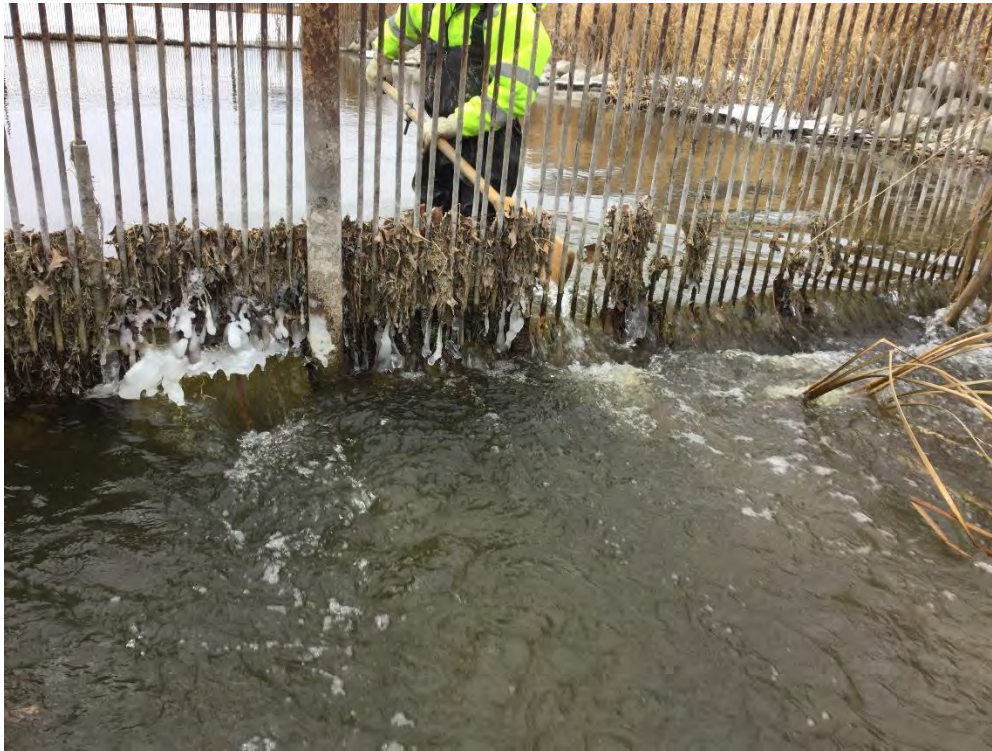
Photo 5: Clearing out the fish barrier improves flow.
